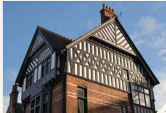
This building demonstrated the virtues of using brick. It is clear from his writings that Allan saw advantages in this as a clean, modern material with a regular form which allowed the development of cavity walling to reduce the possibility of the transmission of dampness to the interior of the building.
